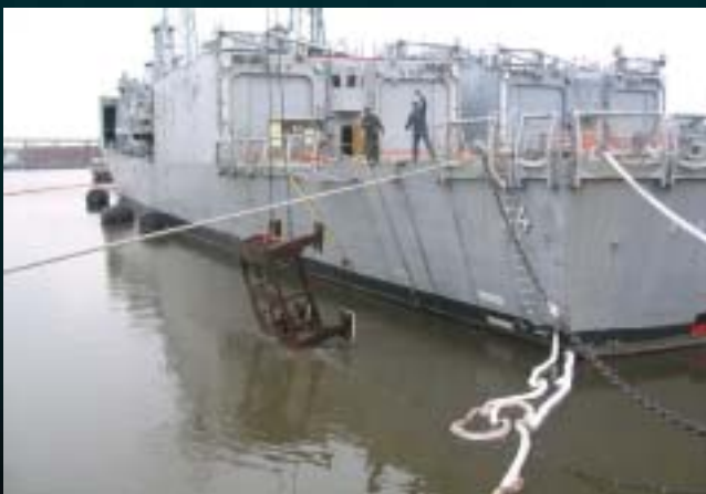
Upper part of Cofferdam structure coming out of the water.
