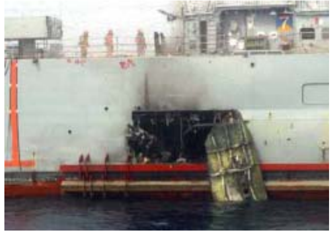
Hull damage from blast. Crack arrestors (external hull stiffeners) were installed previously to limit damage based on pre-test predictions.
