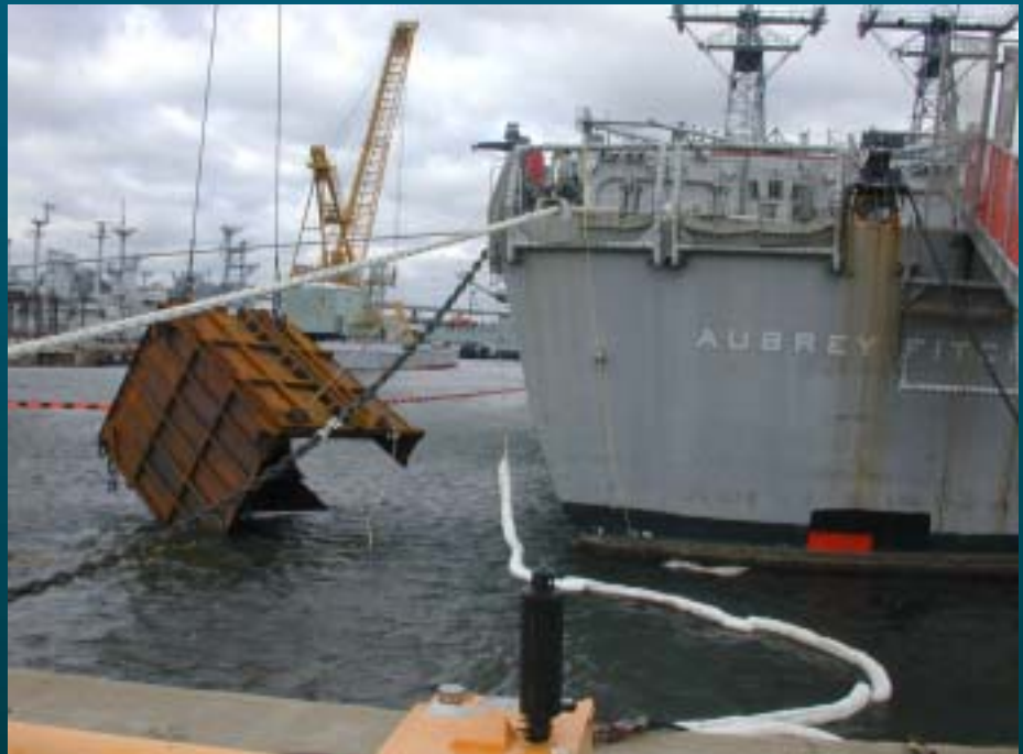
Cofferdam being lowered into place.
