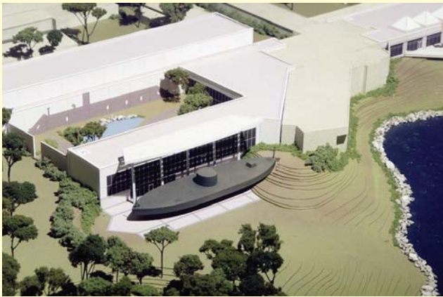
View of the proposed MONITOR Center and its full-scale sculptural replica of the USS MONITOR. Visitors may walk the entire length of the replica's 172-foot deck, giving them a sense of what it would have been like on the original ship.
