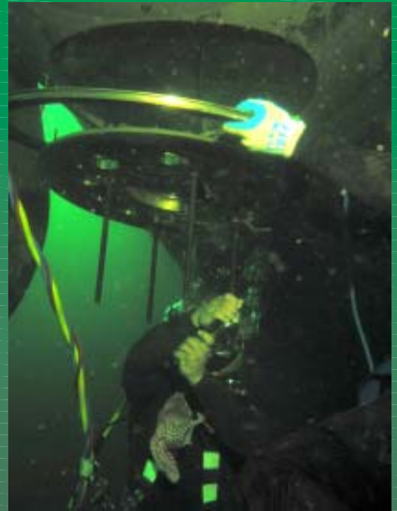
Divers Removing BSBR.
