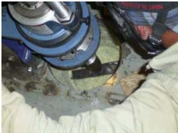
Creating second of two hull cuts.
