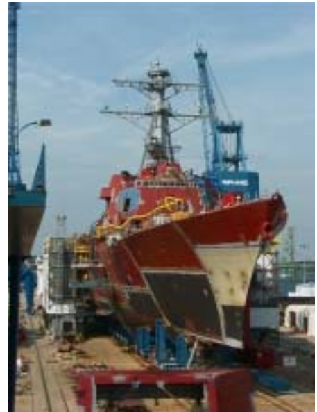
Land Level Ship Construction.
