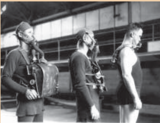
Several variations of the "Momsen Lung" apparatus. Left to right: TM1(DV) Edward Kalinowski in an experimental metal canister, SF1(DV) John Iben in an experimental rubber canister, and LT Charles Momsen in a circular tube around shoulders, March 1928.
