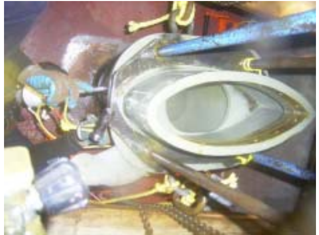
Divers inserting seachest into hull.
