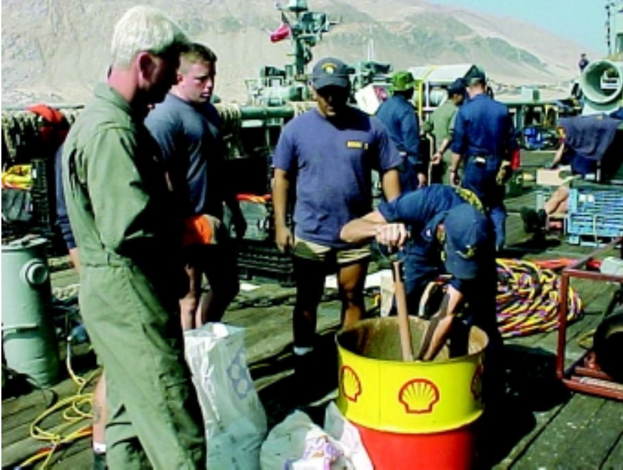
HTC Mike Lutz, GM1 Chad Dillon, SM2 Jorge Guillen, and HT2 Andrew Cowan hand mixing concrete aboard the Chilean Tug, Galvarino.
