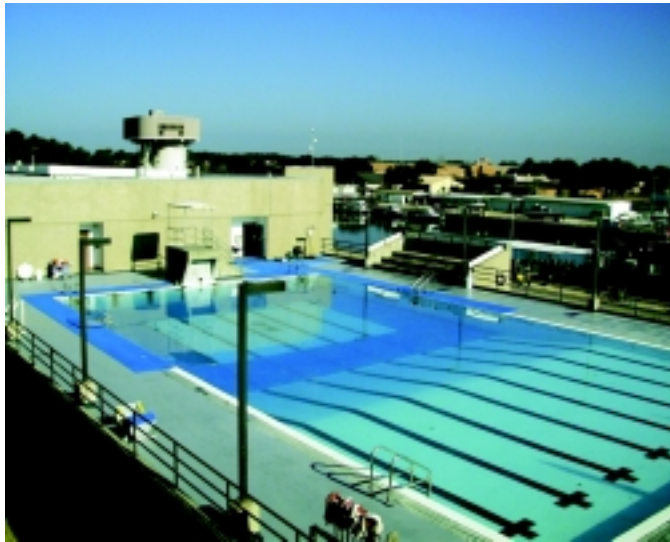
The 33 yard, 12 foot deep, 8 lane dive pool.
